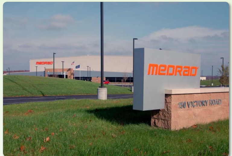
MEDRAD Sterile Disposables Manufacturing Facility
